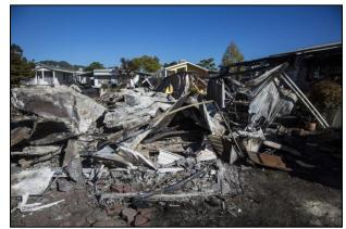
Fire damage from a broken gas line after a Napa Valley Earthquake, August 2014 Source: FEMA
